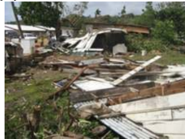
A scene of the damage created by Cyclone Rene on Vava'u, Tonga.
