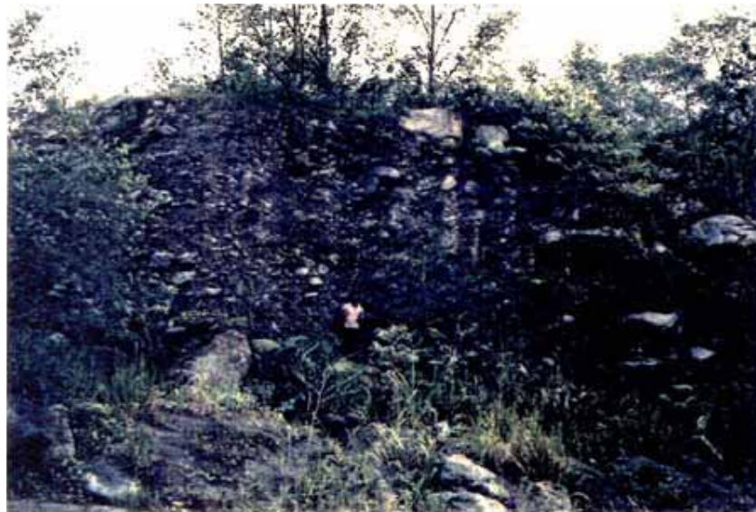
Figure 14. Terrace riser (approximately 8m high) in upper Sutakama watershed. showing large boulders and unsorted nature of deposits. Terrace pre-dates Cyclone Namu. Partly revegetated deposits from Cyclone Namu are visible in foreground.
