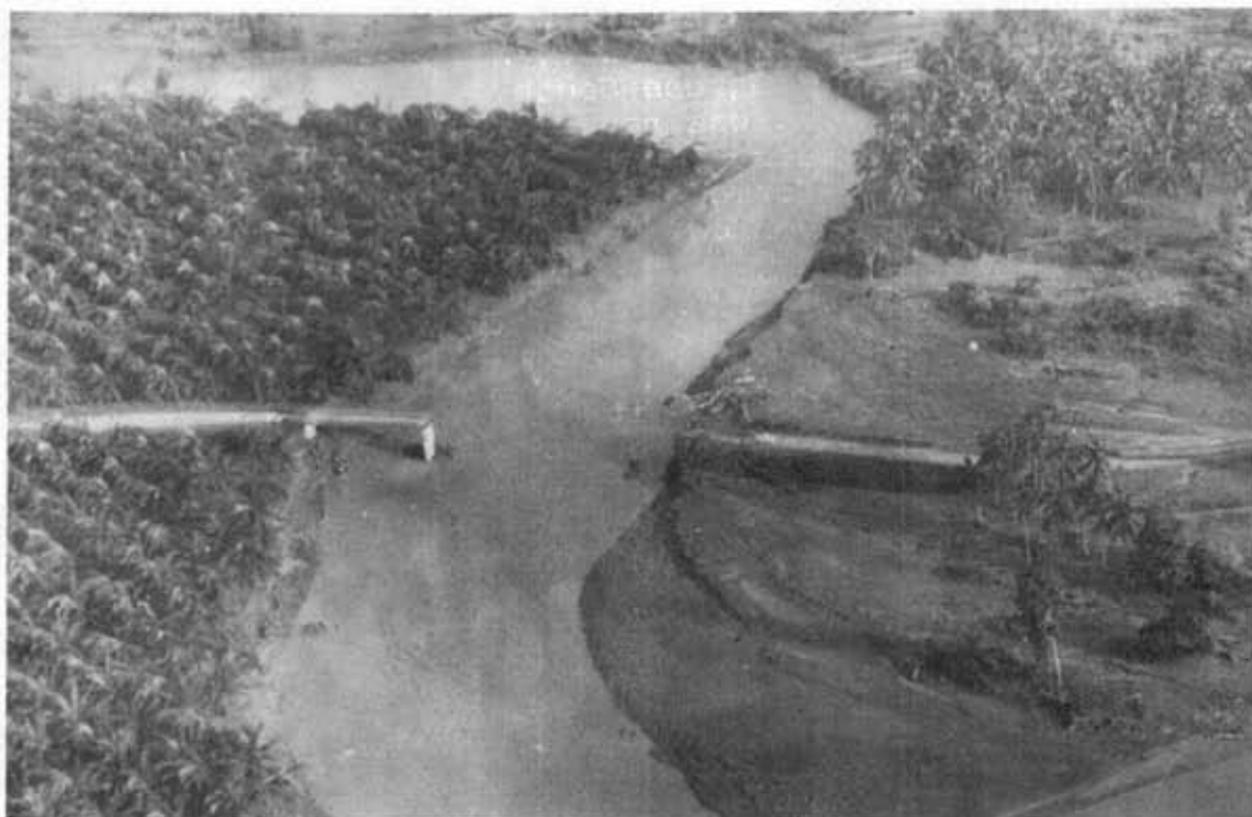
FIGURE 5. THE DEVASTATED MBALISUNA BRIDGE, GUADALCANAL.
