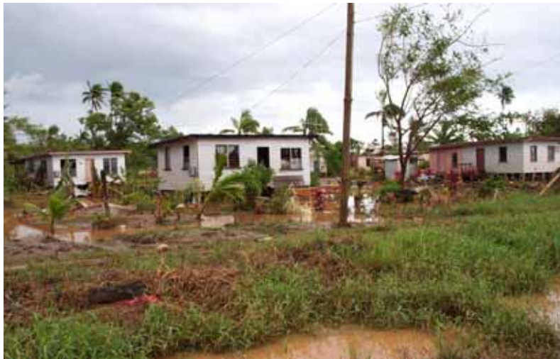
Flooding scar after water receded Photo: Ministry of Information
