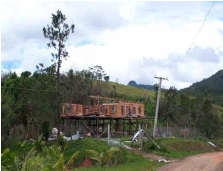
House in ruins after the cyclone
