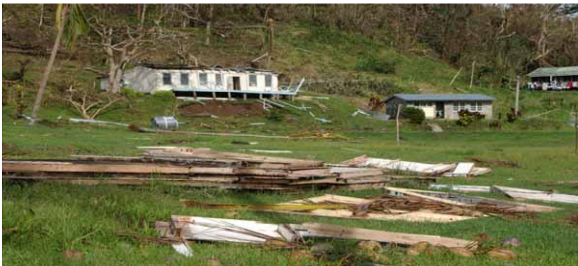
The remains of a damaged building Photo: Fiji Times Ltd
